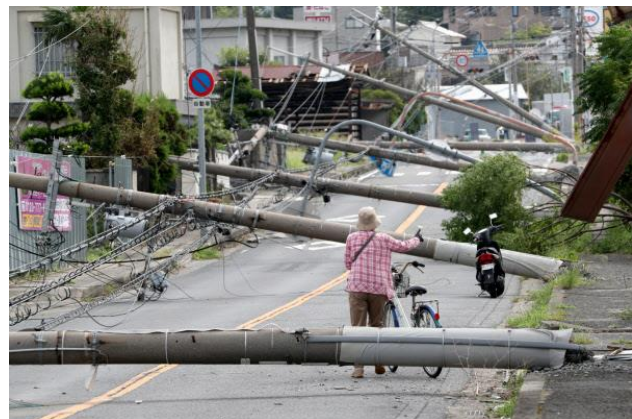
Fig.3 Fallen utility poles blocking a road in Osaka ( https://www.nikkei.com/article/DGXMZ049287500S9A900C1000000/ )
